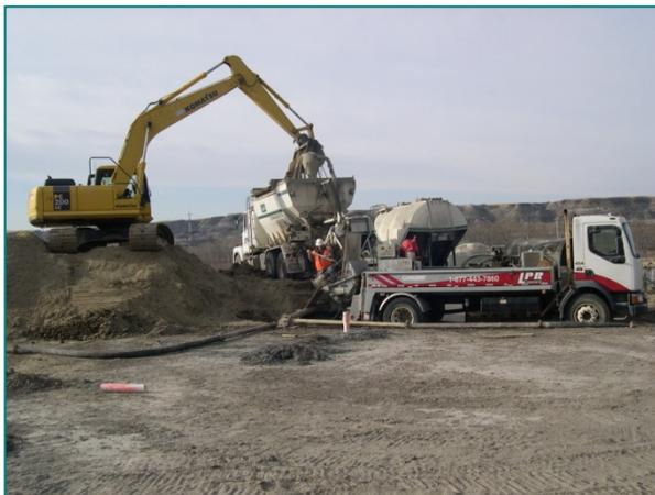
*Mobile Paste Backfill Equipment*
