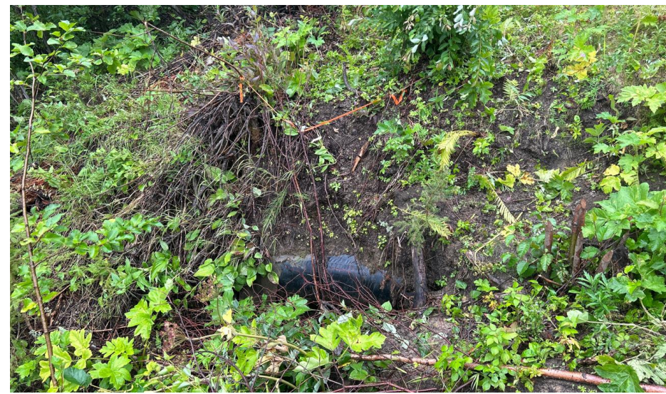
PM-7A Watercourse exposure
