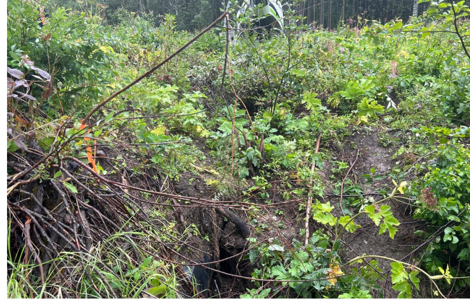
PM-7A Watercourse exposure
