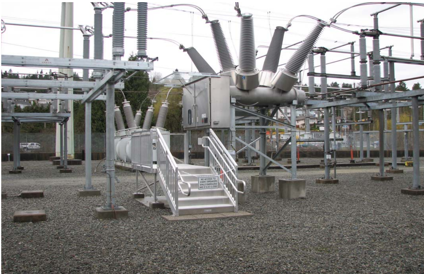
Figure 2. Typical Installation of a 230 kV SF6 Circuit Breaker
