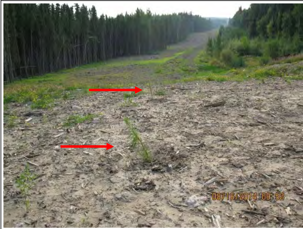
Plate 3 Example of conifer seedling planting on a pipeline right-of-way. The upland area has sufficient drainage and suitable soils for seedling establishment and growth. Photo source: CH2M HILL.
