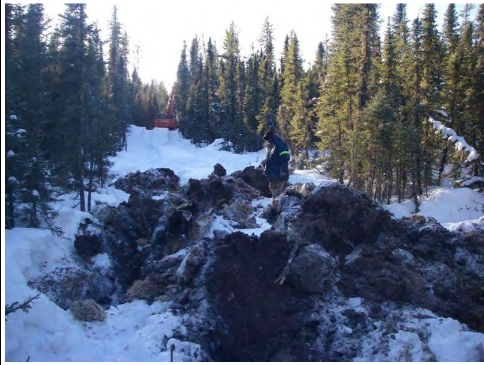
Plate 5 Example of mounding a seismic line. Photo source: Golder 2013, in TERA 2014a.
