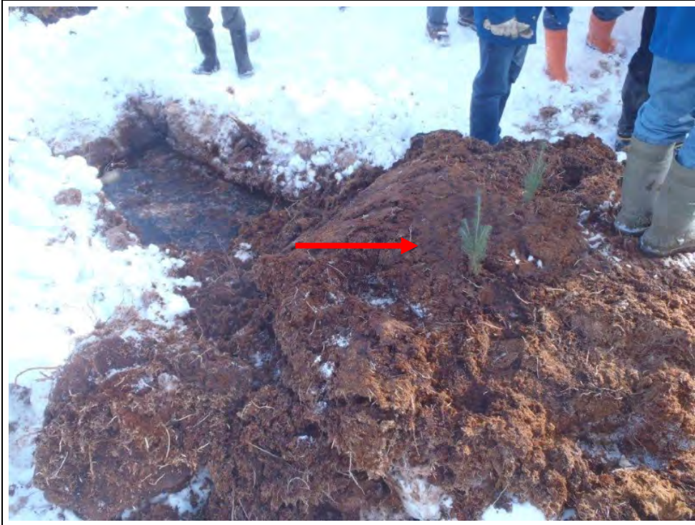
Plate 7 Example of excavator mounding with tree planting. Mounds create microsites that can enhance survival and growth of planted seed and seedlings, and natural regrowth of woody species. It is commonly used in wet, low-lying areas to create better drained microsites for seedlings. Photo source: Golder 2013, in TERA 2014a.
