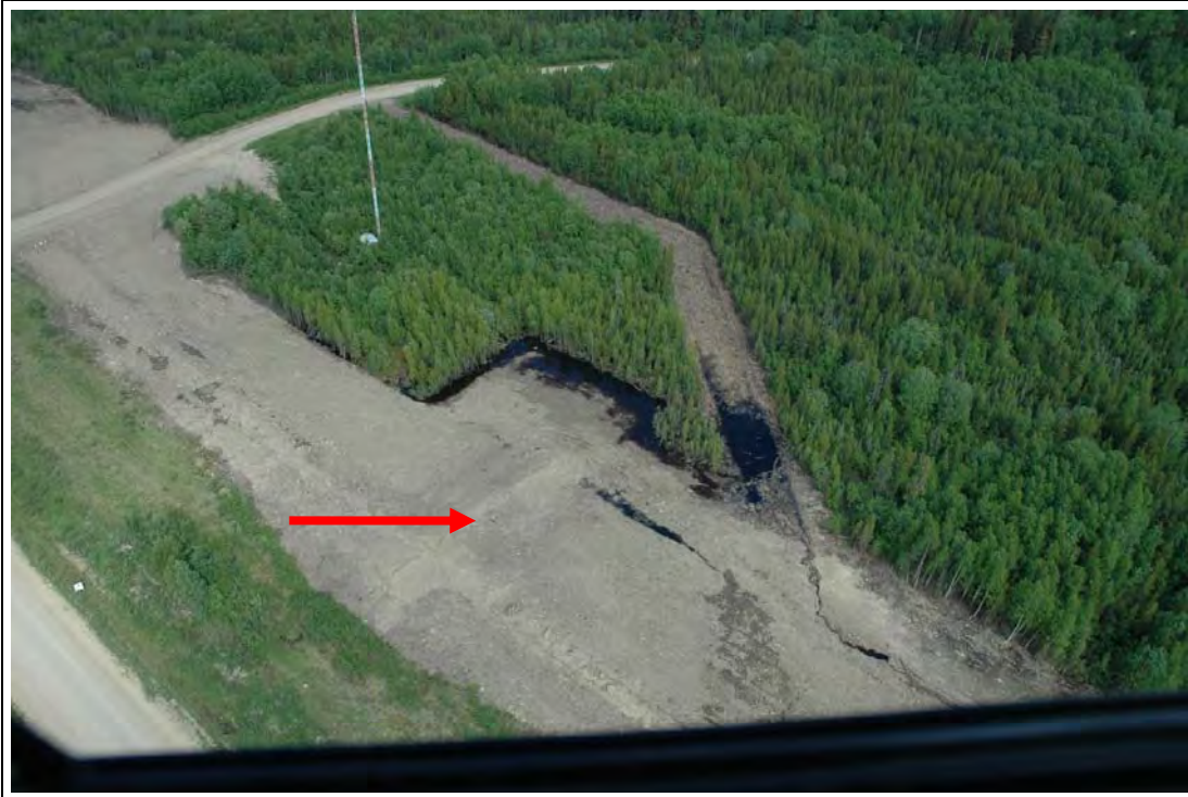
Plate 25 Example of access/line-of-sight management (earth berm) on a new pipeline right-of-way. The measure is unlikely to be effective due to its location relative to existing roads and pipeline right-of-way. Photo source: CH2M HILL.
