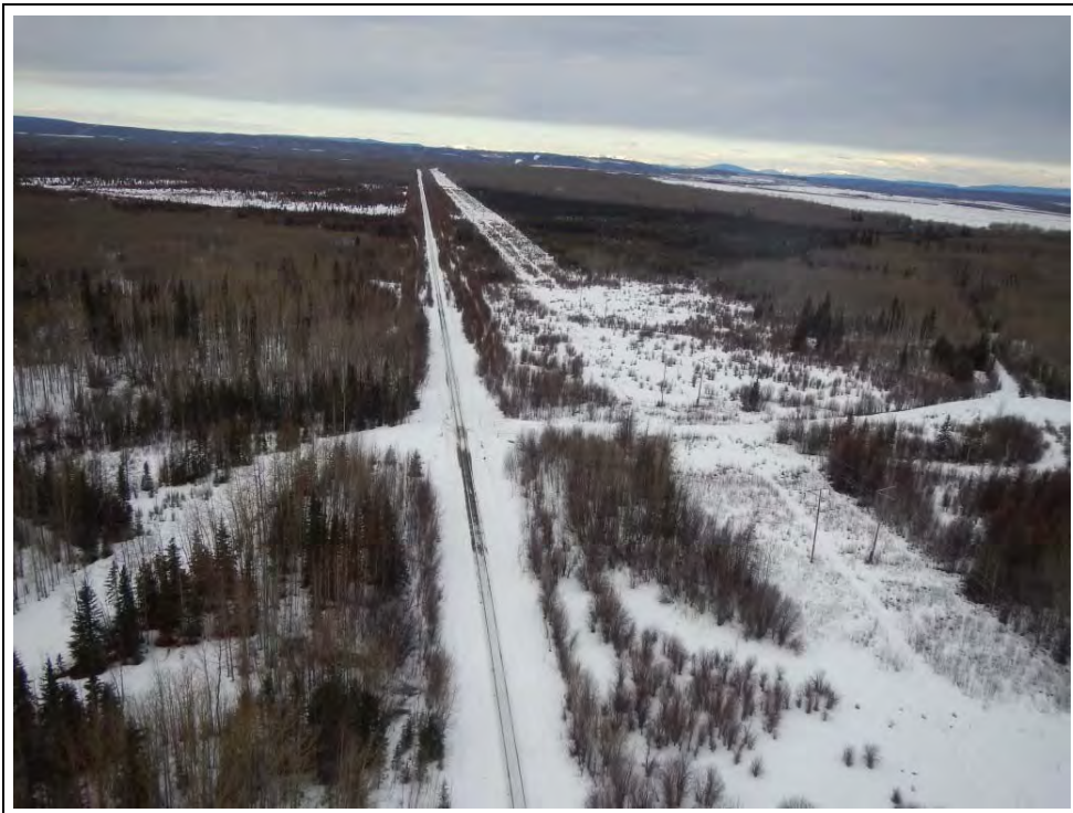
Plate 22 Example of an electrical transmission line paralleling an existing pipeline right-of-way. Where a new pipeline right-of-way parallels an existing linear corridor with multiple rights-of-way, access management would not be effective. Photo source: CH2M HILL.
