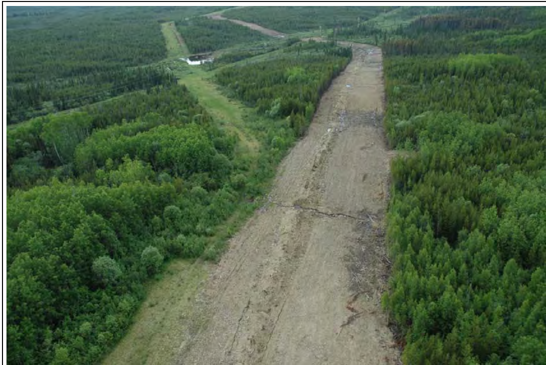
Plate 8 Example of a vegetation screen retained along edge of pipeline right-of-way at intersection with an existing linear disturbance. Vegetation screens block line-of-sight and can effectively manage access. Photo source: CH2M HILL.
