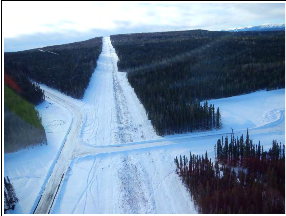
Plate 23 Example of multiple existing linear disturbances that facilitate access (plowed roads, pipeline right-of-way). Access management on a new paralleling pipeline right-of-way would be ineffective. Photo source: CH2M HILL.
