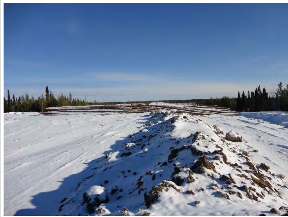
Plate 9 Example of a wood berm to deter access and reduce line-of-sight. To effectively block line-of-sight, berms should be constructed to an approximate minimum height of 1.5-2 m. Alternate measures are preferred over berms given the multiple limitations and low value. Value may be improved with shrub planting at base of berm and extending into adjacent forest. Photo source: NGTL.
