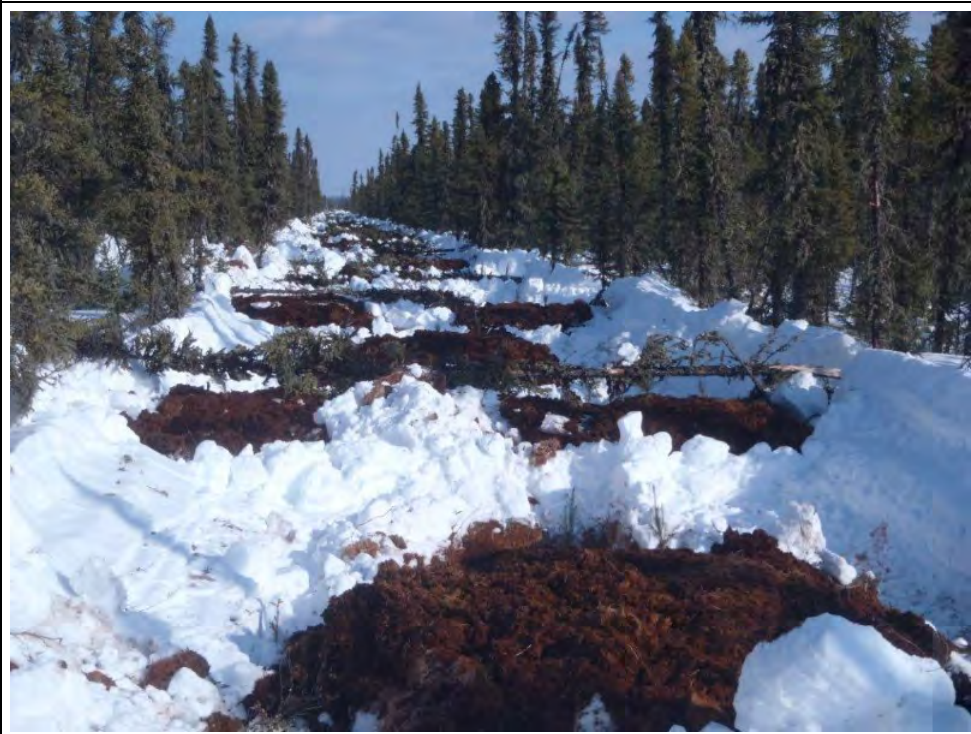
Plate 6 Example of mounding combined with tree-felling and conifer seedling planting on a seismic line. The combination of measures (often referred to as “line-blocking”) is intended to manage human and predator access, and facilitate revegetation of conifers. Photo source: Golder 2013, in TERA 2014a.
