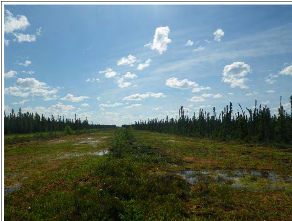
Plate 20 Example of multiple rights-of-way in a tree fen. Regrowth of vegetation can be limited by soil temperature, drainage and nutrients. Line-of-sight breaks and access management measures are ineffective in locations such as this. Minimum disturbance construction during frozen conditions (including ramp overs) are typically the preferred option for enhancing restoration. Photo source: CH2M HILL.
