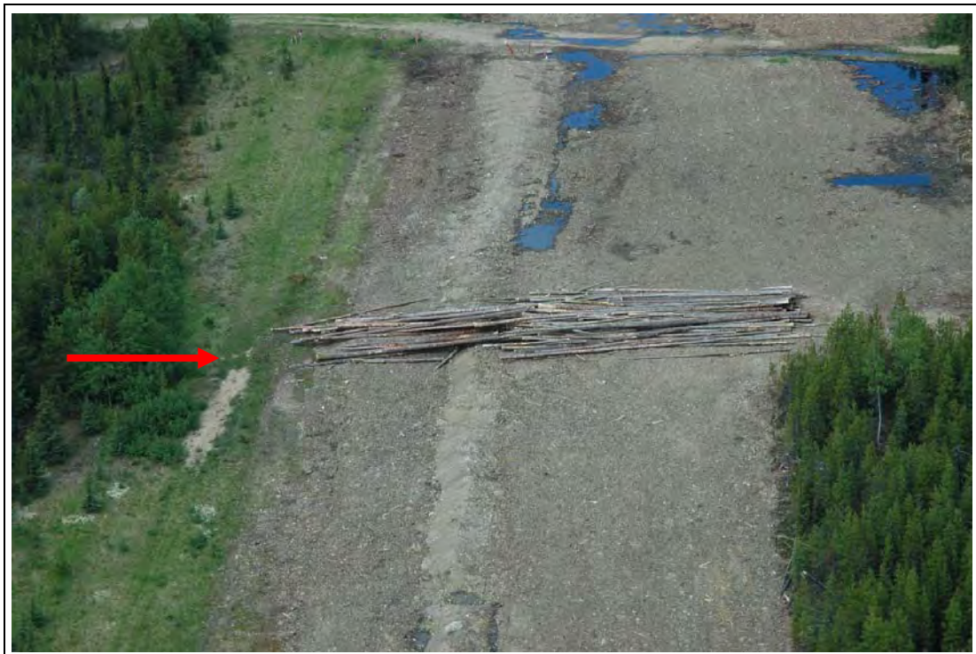
Plate 24 Example of access management (wood berm) on a new paralleling pipeline right-of-way that would be ineffective due to existing linear disturbances that facilitate access. Photo source: CH2M HILL.
