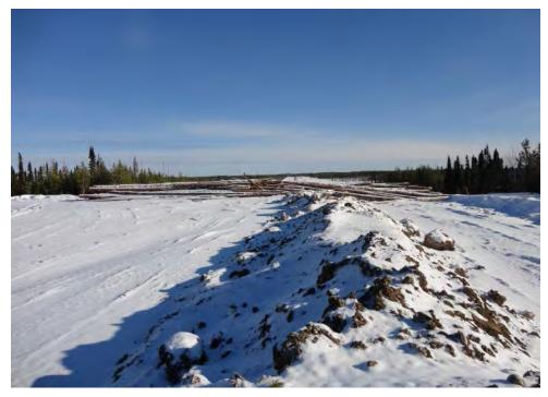
Plate 7: Example of a wood berm designed to deter access and reduce line-of-sight. This measure is no longer used due to the risks associated with forest fires. Photo source: NGTL.
