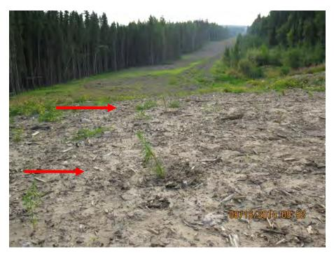
Plate 3: Example of conifer seedling planting on a pipeline ROW. The upland area has sufficient drainage and suitable soils for seedling establishment and growth. Photo source: CH2M HILL.
