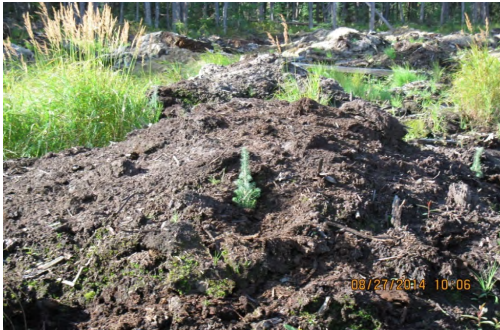
Plate 11: Example of mounding combined with conifer seedling planting on a ROW. The combination of measures is intended to manage access, and facilitate revegetation of conifers. Photo source: NGTL.
