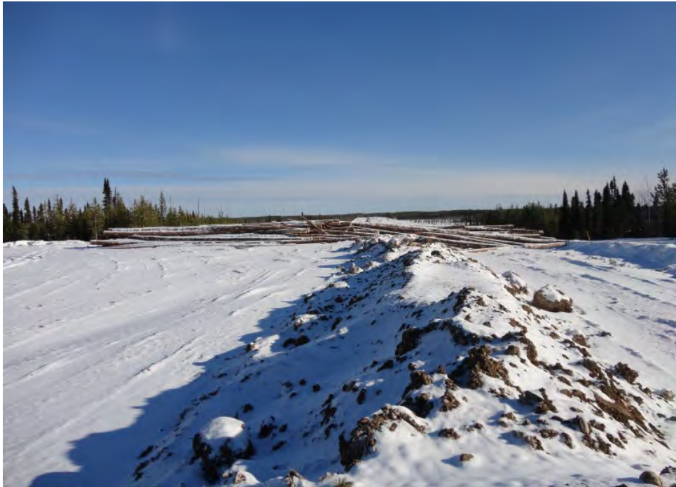
Plate 7: Example of a wood berm designed to deter access and reduce line-of-sight. This measure is no longer used due to the risks associated with forest fires. Photo source: NGTL.
