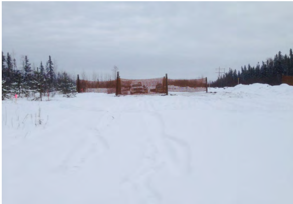
Plate 10: Fabricated line-of sight on a ROW paralleled by another ROW and a power line. This measure is not fully effective due to the presence of adjacent developments where no line-of-sight measures are implemented. Photo source: NGTL.
