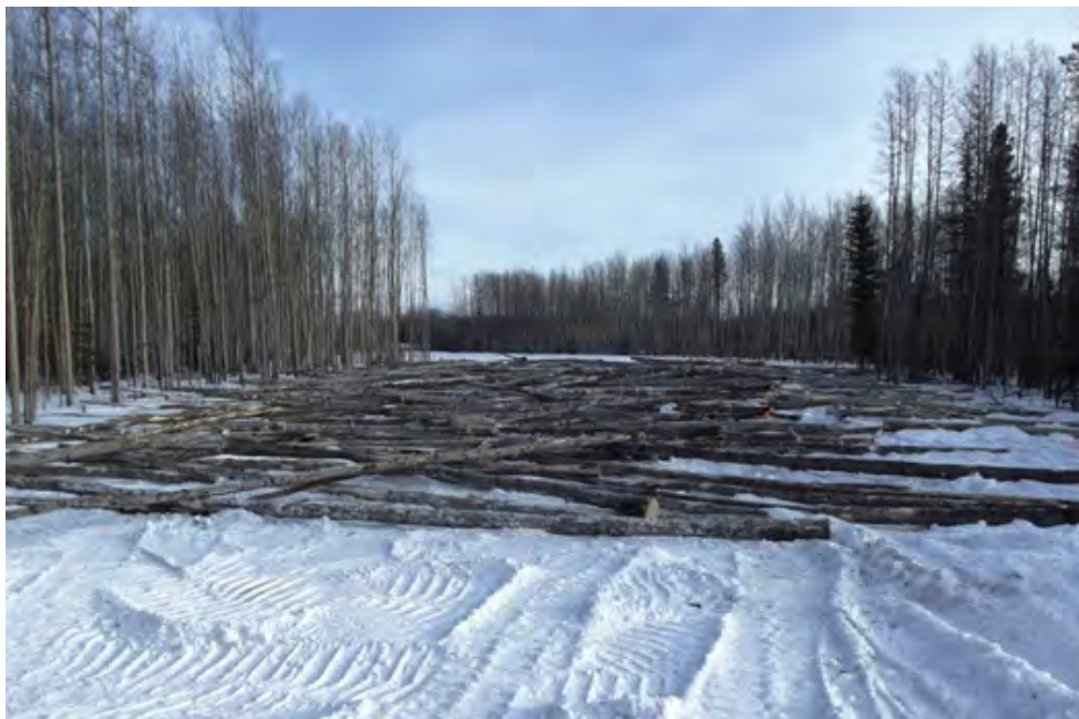
Plate 2: Example of coarse woody debris rollback for access management on a non-parallel pipeline ROW. The debris also creates microsites to enhance vegetation establishment and growth. Photo source: NGTL.
