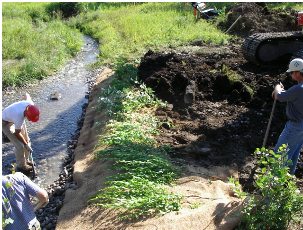
Plate 12: Example of shrub staking in the riparian area at a watercourse crossing. Photo source: NGTL.
