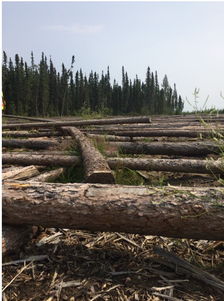
Plate 13: Example of lattice placement of rollback. Photo source: NGTL.
