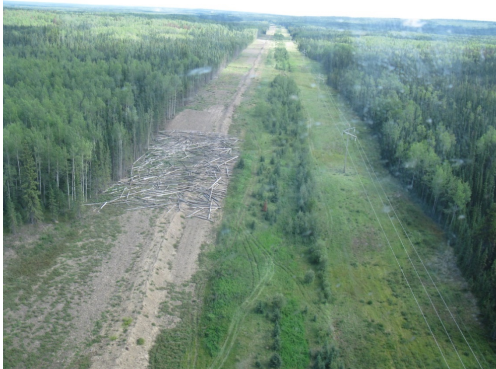
Plate 4: Example of access management implemented on a ROW with parallel developments. Note the ATV tracks that divert around the woody debris rollback. Photo source: NGTL.
