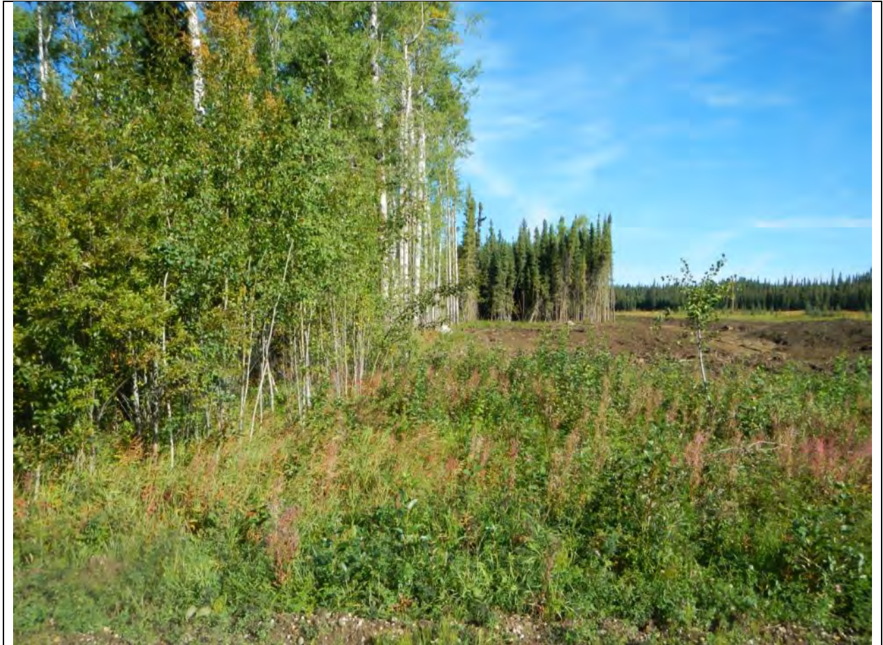
Figure 5 Example of Minimum Disturbance Construction, Hand-Cutting of Vegetation along a Pipeline ROW, at a Road Intersection
