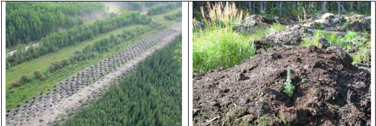
Figure 4 Example of Mounding along a Pipeline ROW from the Air (left) and Ground (right)
