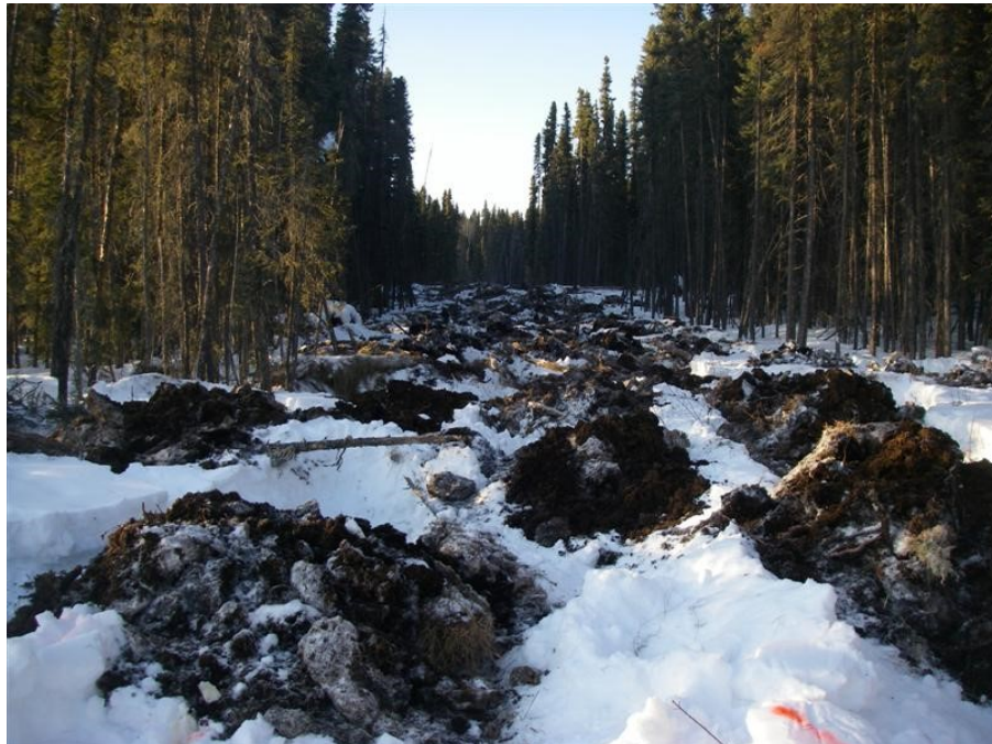
Plate 4: Example of mounding used as an access management measure and to facilitate caribou habitat restoration through the creation of microsites that improve vegetation establishment. The treated linear disturbance is a seismic line, which is substantially narrower than a pipeline right-of-way. Photo source: Golder 2013, in TERA 2014.
