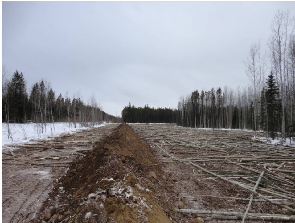
Plate 2: Example of coarse woody debris rollback for access management on a pipeline right-of-way. The debris also creates microsites to enhance vegetation establishment and growth. The trench material has not yet settled in this photo. Photo source: NGTL.
