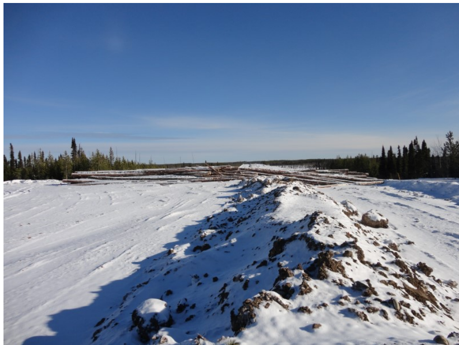
Plate 6: Example of a wood berm to deter access and reduce line-of-sight. To effectively block line-of-sight, berms should be constructed to an approximate minimum height of 1.5-2 m. Alternate measures are preferred over berms given the multiple limitations and low value. Value may be improved with shrub planting at base of berm and extending into adjacent forest. Photo source: NGTL.
