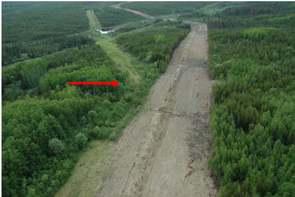
Plate 10: Example of a vegetation screen retained along edge of pipeline right-of-way at intersection with an existing linear disturbance. Vegetation screens block line-of-sight and can effectively manage access. Photo source: CH2M HILL.
