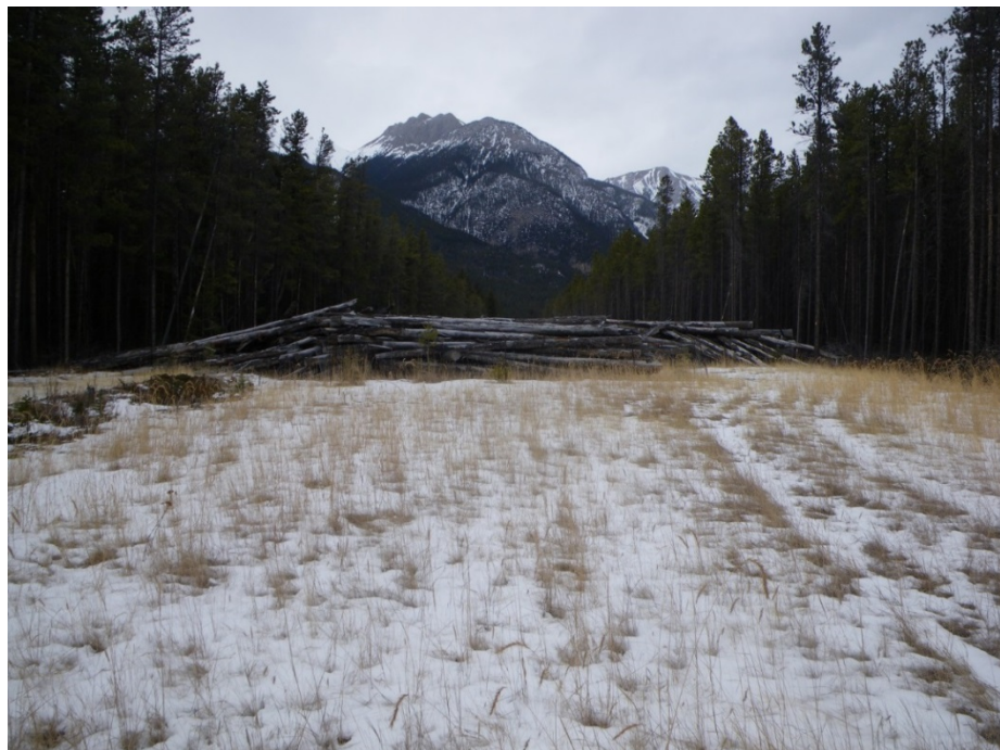
Plate 8: Supported woody debris berms resemble log fences or walls, constructed using timber cleared from the right-of-way. Limitations to supported berms include availability of material, ability of the soils to support the structure, and whether the right-of-way is adjacent to an existing linear disturbance that cannot be blocked. Photo source: CH2M HILL.
