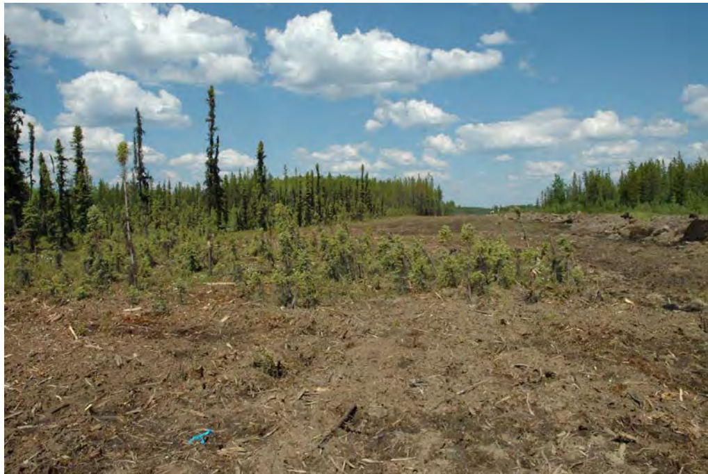
Plate 11: Example of a ramp-over area where a snow ramp was packed over vegetation in a treed lowland. The resultant vegetation screen will contribute to natural regeneration on the adjacent areas of the footprint. Site conditions and construction requirements can limit the use of this measure. Photo source: CH2M HILL.
