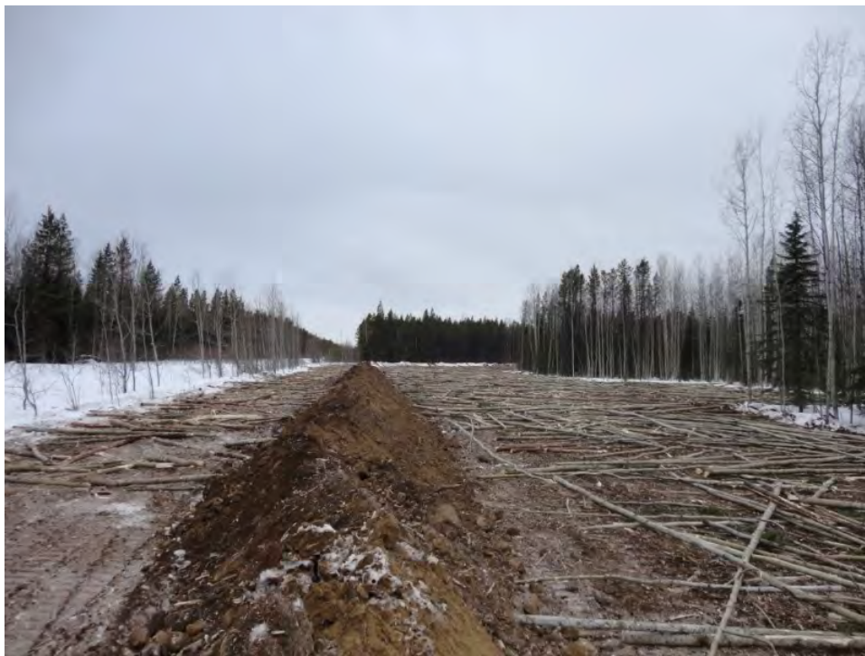
Plate 2: Example of coarse woody debris rollback for access management on a pipeline right-of-way. The debris also creates microsites to enhance vegetation establishment and growth. The trench material has not yet settled in this photo. Photo source: NGTL.
