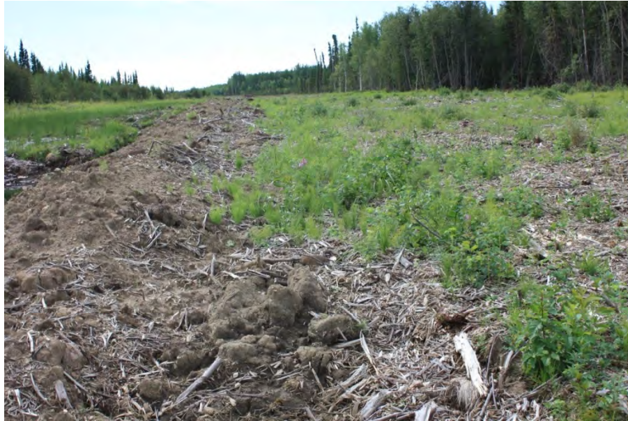
Plate 13: Example of natural regeneration during the first growing season following pipeline construction in an upland/transitional site where minimum disturbance construction was implemented. Natural regeneration of alder, willow, rose, and various forbs is evident. Natural regeneration was supplemented with white spruce seedling planting in this location. Photo source: CH2M HILL.
