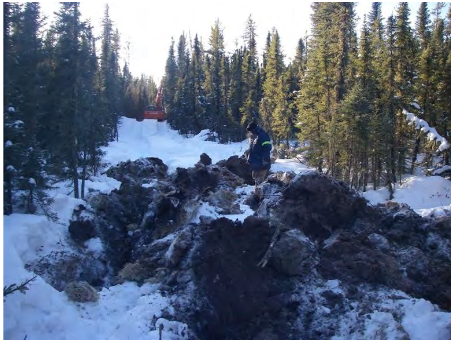
Plate 5: Example of mounding a seismic line. Photo source: Golder 2013, in TERA 2014.
