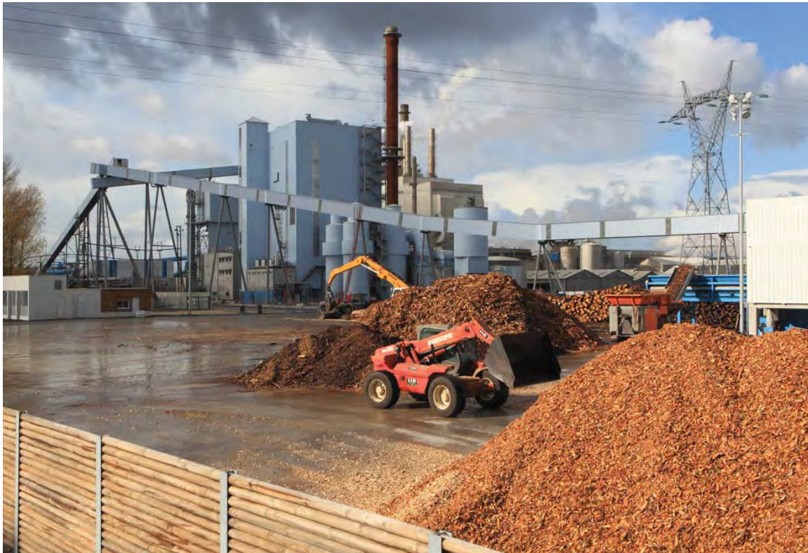
Figure 48: 50 MW biomass bubbling fluidized bed plant located in France
