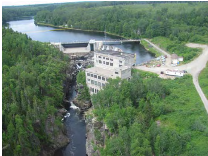
Figure 28: NB Power's existing Nepisiguit Falls Generating Station
