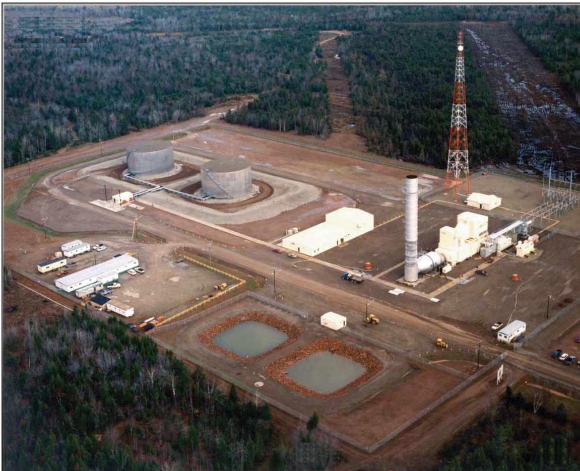
Figure 58: The Ste. Rose Generating Station
